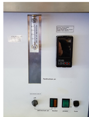
New flow meter & controller as part of the upgrade
