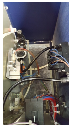
View of upgraded FB08 controls
